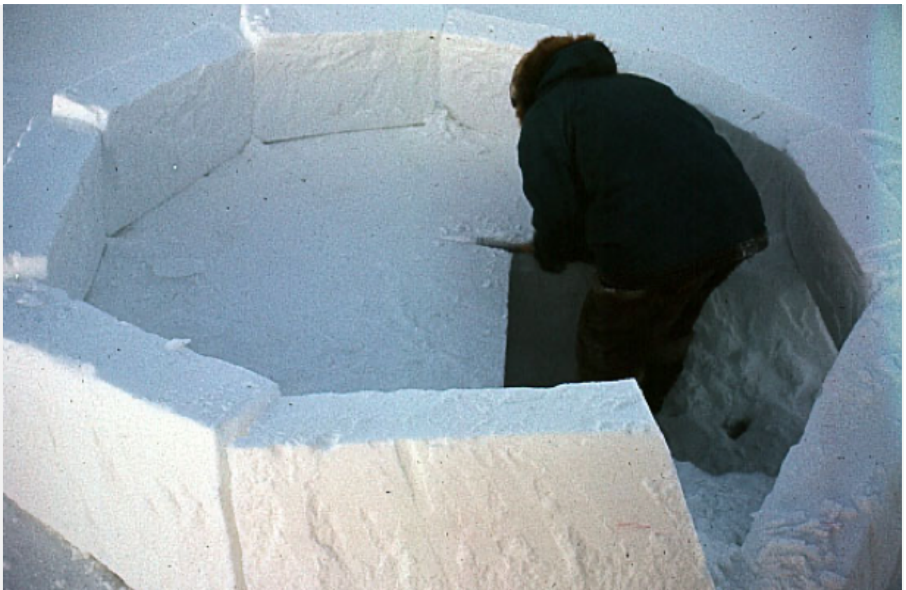
Tipana demonstrates the secret of successful Igloo construction by placing his snow blocks ‘one-on-one’ in a spiral (Colin Irwin — Arctic Trek 1973)
